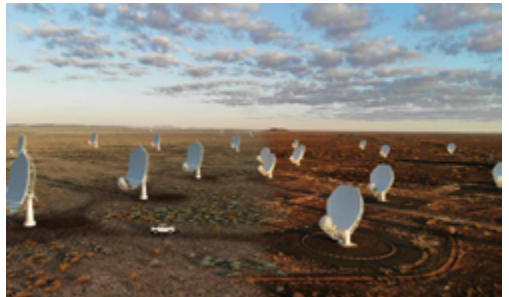
Figure 2: Artistic impression of the future SKA-Mid telescope, which is composed of many individual telescopes distributed over a large area. Note that radio waves can be received also during day time and through cloudy skies, in contrast to optical waves from outer space. © Square Kilometre Array Observatory, 2021.
